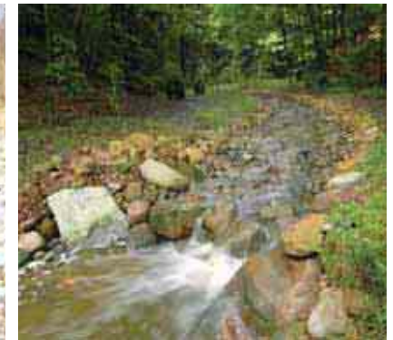
Constructed steppool will restore stream to grade
